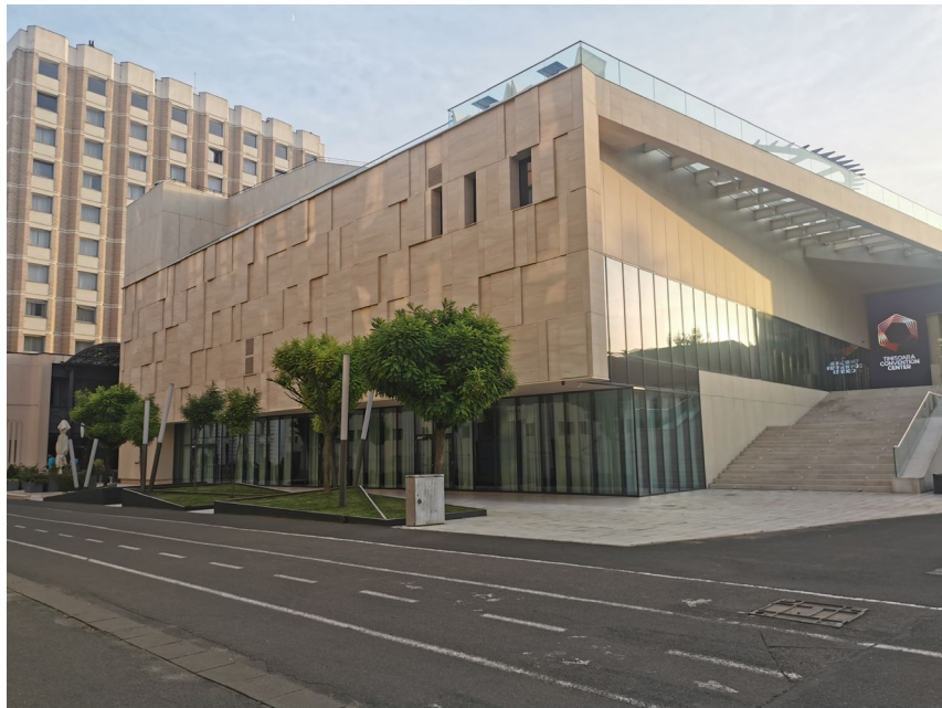
Marasesti Street, view from the main entrance - Hotel Timisoara.
